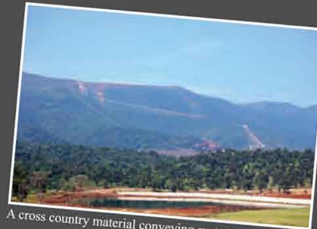
A section of a Coal Handling Plant (CHP)
