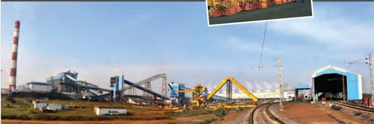
TRF's processing system and equipment in a power plant
